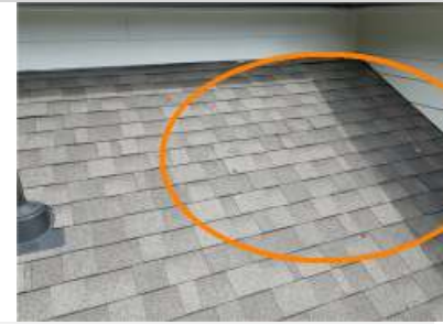
Item 8 - Item 12 (Picture) Example - Item 3 - Evidence of foot traffic
