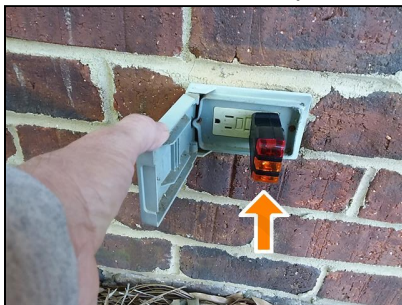
The left exterior GFCI electrical outlet did not trip when tested, investigate.
