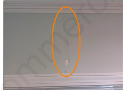
hallway, settling crack, repair, investigate
