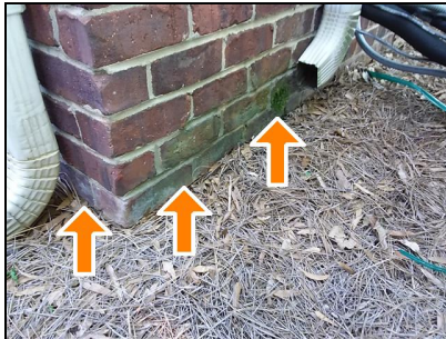
left rear exterior, efflorescence and moisture on the wall, gutter needs splash block, investigate
