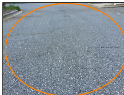
asphalt parking lot, cracks seal, investigate
