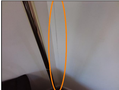
Office 2, sheetrock tape coming loose, repair, investigate
