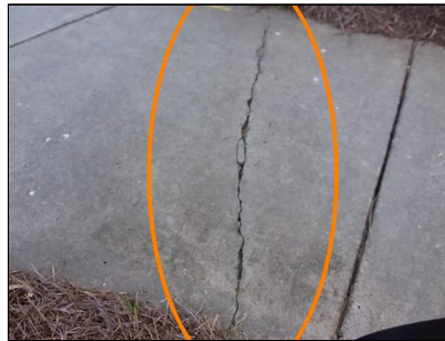
front exterior, crack seal, investigate
