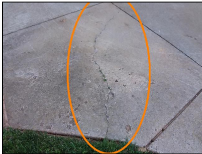
rear exterior, crack seal, investigate
