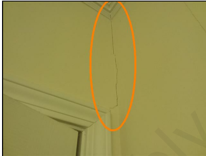
office three, settling crack, repair, investigate
