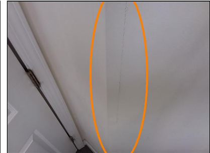
office three, settling crack, repair, investigate
