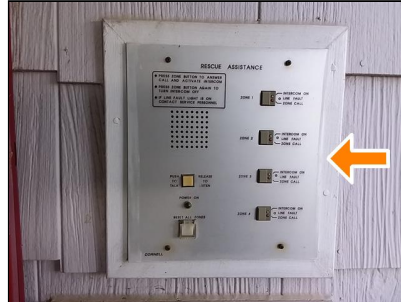
front exterior, rescue assistance control panel
