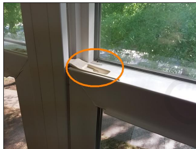
office three, bad clip, repair, investigate
