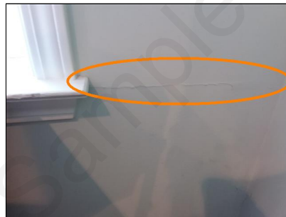
front suite, settling crack, repair, investigate
