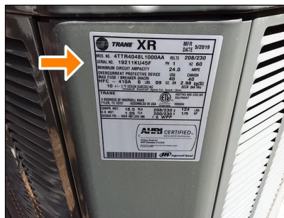
left exterior, HVAC unit information, 5/2019
