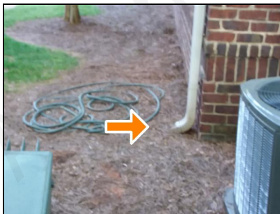
left exterior, splash block needed for gutter, investigate
