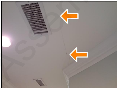
common hallway, settlement crack in ceiling, repair, investigate
