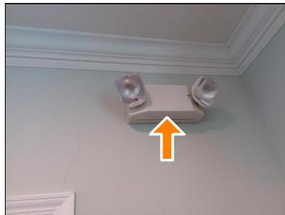
The wall mounted emergency light at the front area did not operate when tested, repair, investigate.
