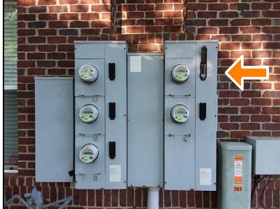
left exterior, main electrical meter and breaker, 100 amp
