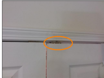
The right top of the door is not latching in office 2, repair, investigate.
