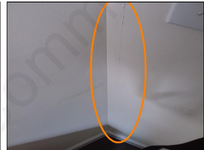
Office 3, sheetrock tape coming loose, repair, investigate
