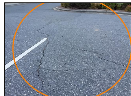
asphalt parking lot, cracks seal, investigate
