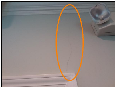
front suite, settling crack, repair, investigate
