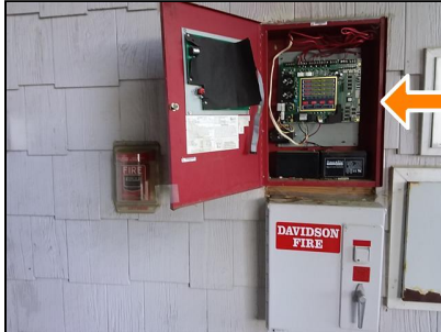
front exterior, FCI fire alarm panel
