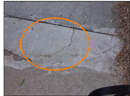
front exterior, crack seal, investigate
