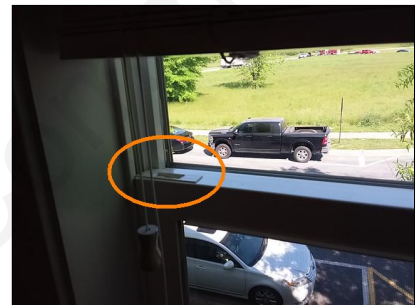
front suite area, bad clip, repair, investigate
