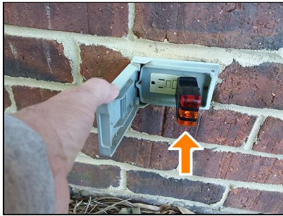
The left exterior GFCI electrical outlet did not trip when tested, investigate.
