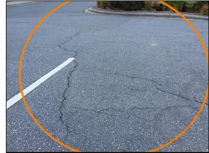
asphalt parking lot, cracks seal, investigate
