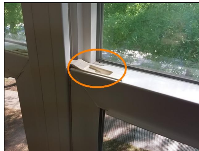
office three, bad clip, repair, investigate
