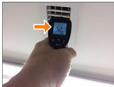
709 suite supply cool air temperature
