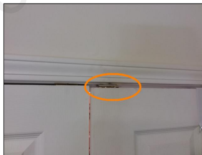
The right top of the door is not latching in office 2, repair, investigate.
