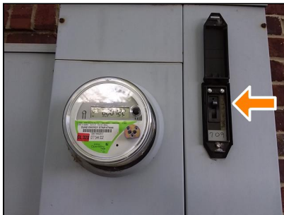
left exterior, main electrical breaker and meter
