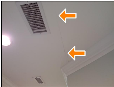
common hallway, settlement crack in ceiling, repair, investigate
