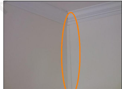
Office 2, sheetrock tape coming loose, repair, investigate
