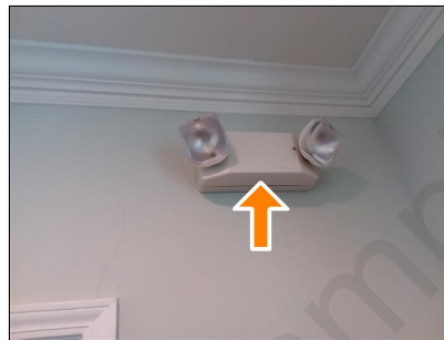
The wall mounted emergency light at the front area did not operate when tested, repair, investigate.
