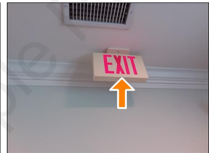
The emergency light above the front door did not operate when tested, repair, investigate.
