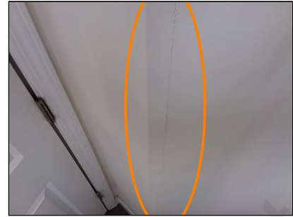
office three, settling crack, repair, investigate
