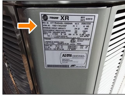
left exterior, HVAC unit information, 5/2019
