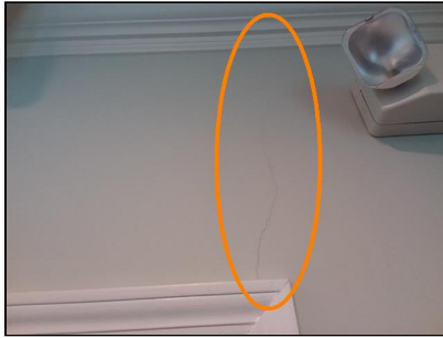
front suite, settling crack, repair, investigate
