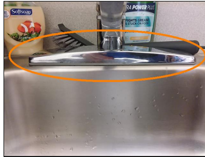
kitchen, sink hardware needs to be secured to the sink pan, repair, investigate
