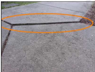
front exterior, trip hazard, repair, investigate
