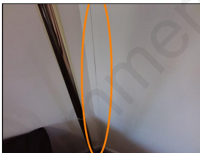
Office 2, sheetrock tape coming loose, repair, investigate
