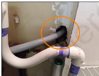
office four closet, seal hole in wall, investigate
