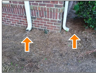
left exterior, splash block needed for gutters, investigate
