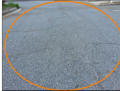
asphalt parking lot, cracks seal, investigate
