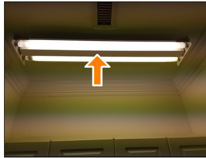
The light fixture in the kitchen ceiling needs a lens cover, repair, investigate.
